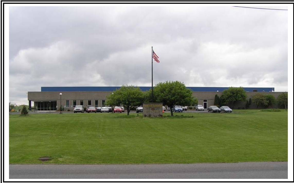
Photo 1, Erie Boulevard, Department of General Services Building
