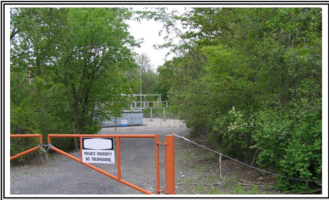
Photo 10, Site 7- Krumkill Road- Niagara Mohawk Substation
